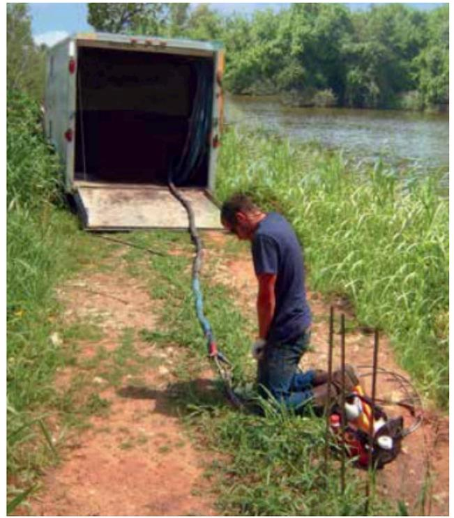
URETEK technician injects structural polymer to create an underground curtain.
