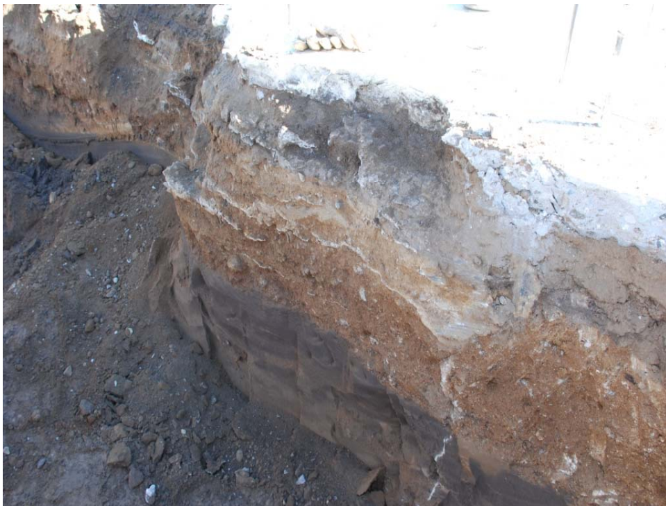
Excavation revealing polyurethane compacting backfill test material and filling voids
