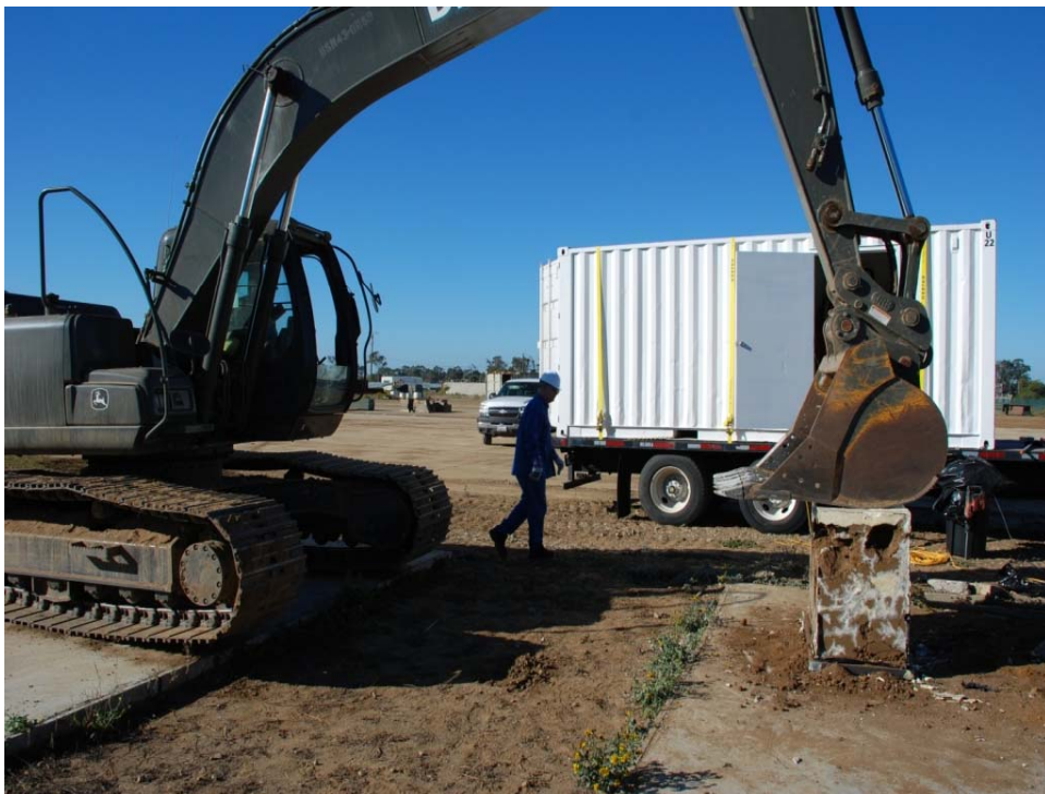
Vertical load applied using an excavator
